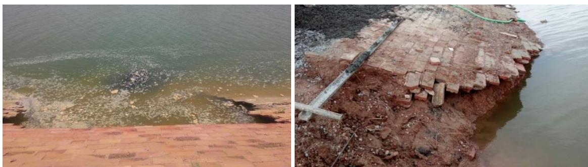
As the flow in the canal is not to be reduced or stopped, conventional strengthening measures in the vulnerable stretches cannot be applied. Any repairing or strengthening activity, particularly for the section below water level needs to be carried out under flowing water condition.
