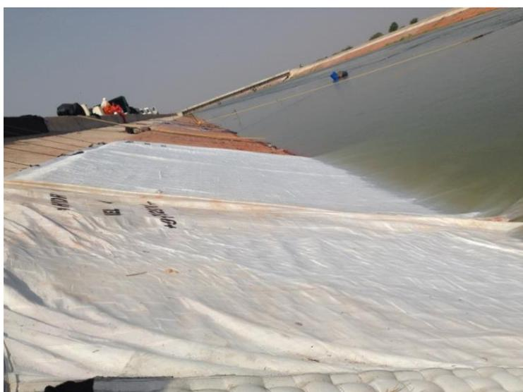
After the canal slopes and bed are cleaned, dressed and leveled, non-woven geotextile and uniform form fabric section was laid with the help of divers. Panels was connected by zipper and hand-held stitching machine. Anchoring was needed prior to filling the concrete grout in to the fabric form to prevent the sliding of panels into canal.
